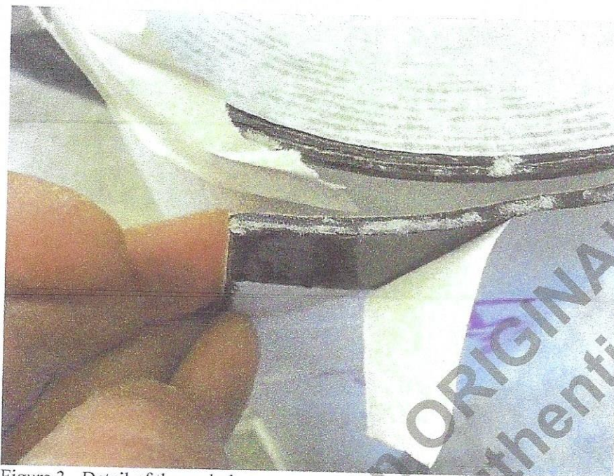
Figure 3 - Detail of the underlayment.
