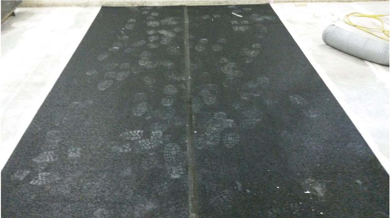
Figure 3 – Detail of underlayment installed on concrete slabs.
