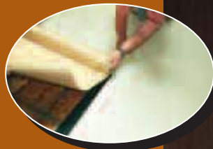
Align with 2" Overlap Remove Paper and Press into Place
