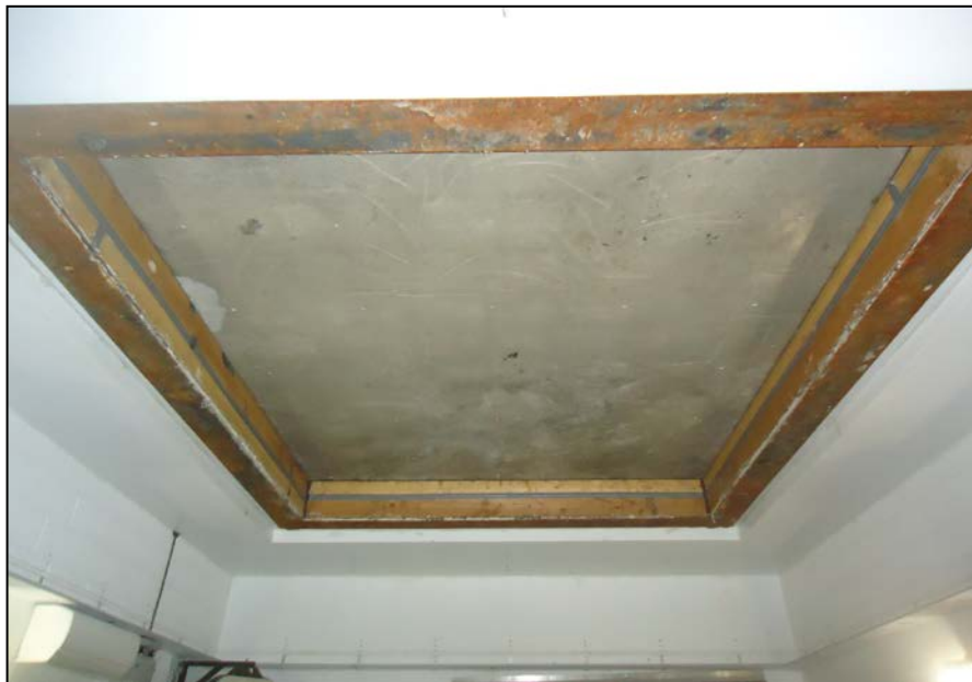
Receive Room View of Test Specimen Installation
